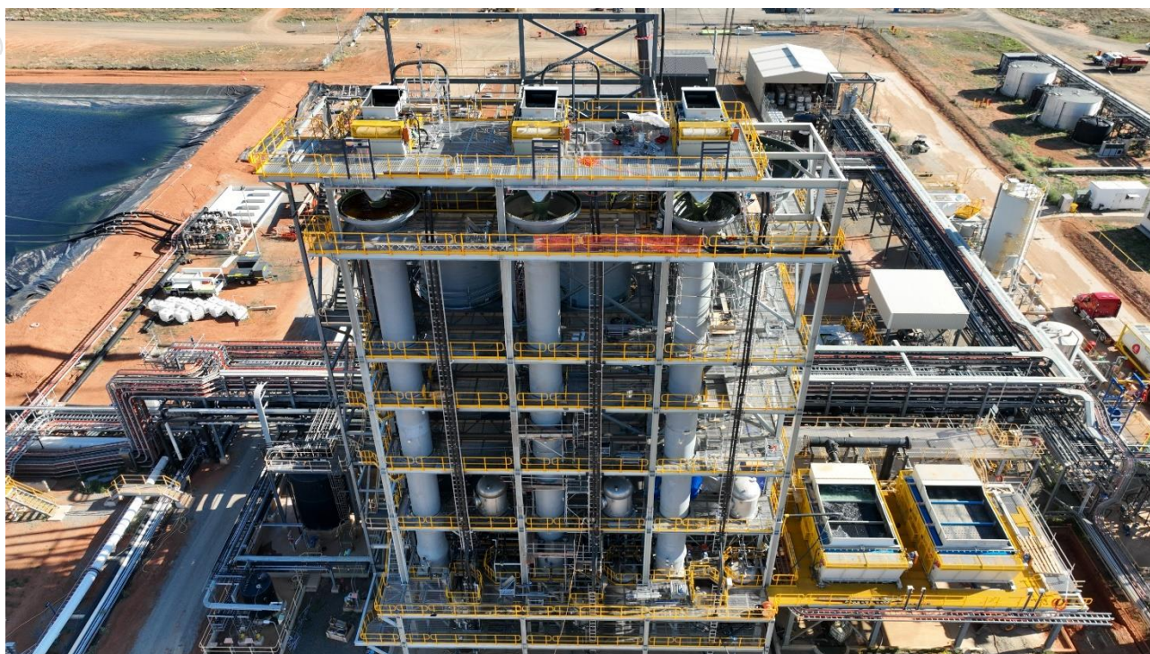
Figure 1: From left to right, NIMCIX columns 1, 2 and 3
