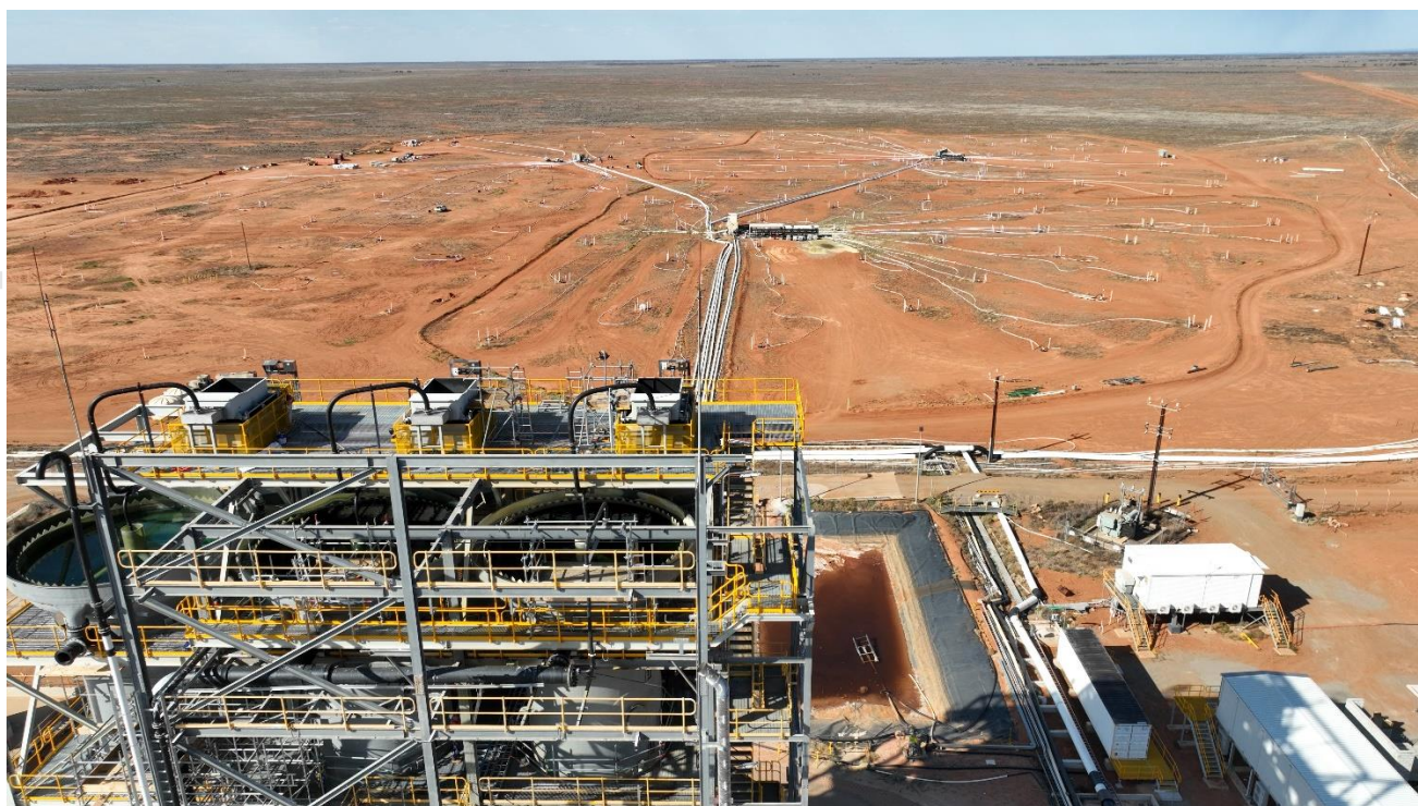
Figure 2: Wellfields 1 and 2 in operation
