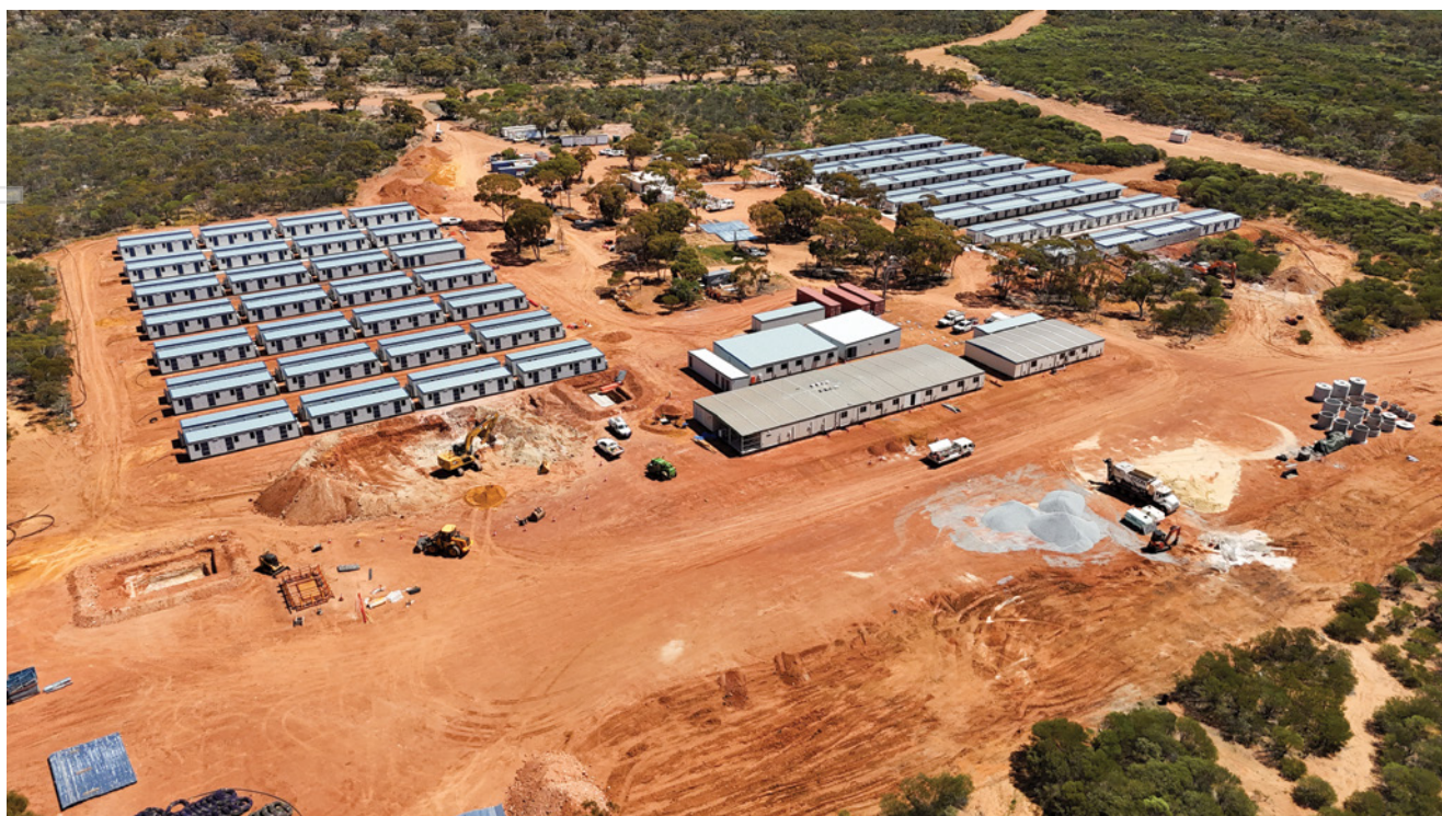
Mt Gibson Gold Project – accommodation village installation
