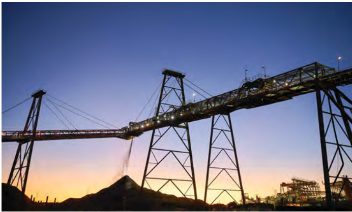
Ernest Henry processing plant and stockpile
