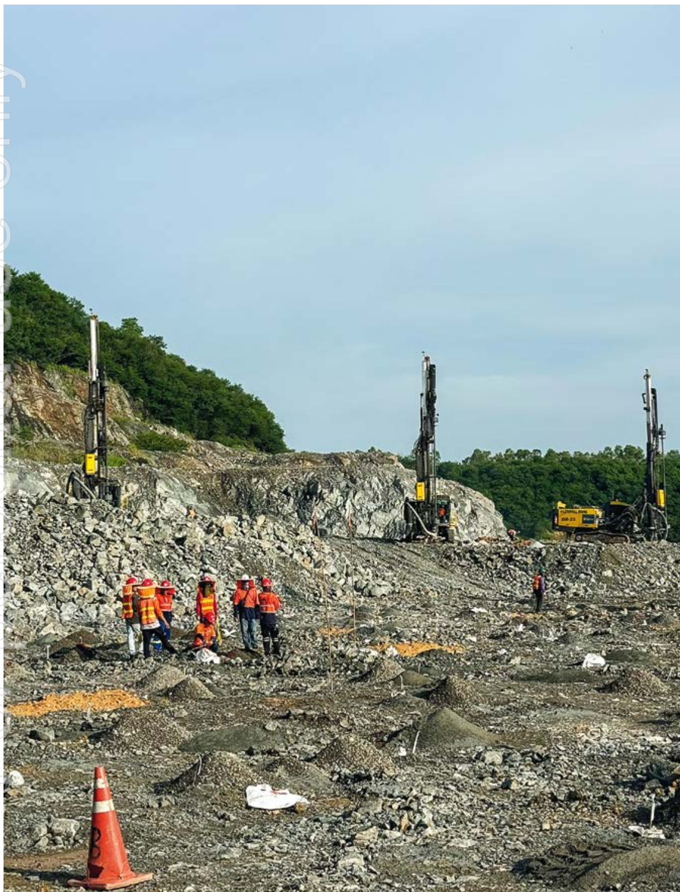
Drill and Blast – A Pit
