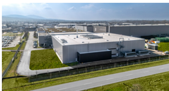
Figure 4 – Mercedes-Benz LiB Recycling Building, Kuppenheim Germany
