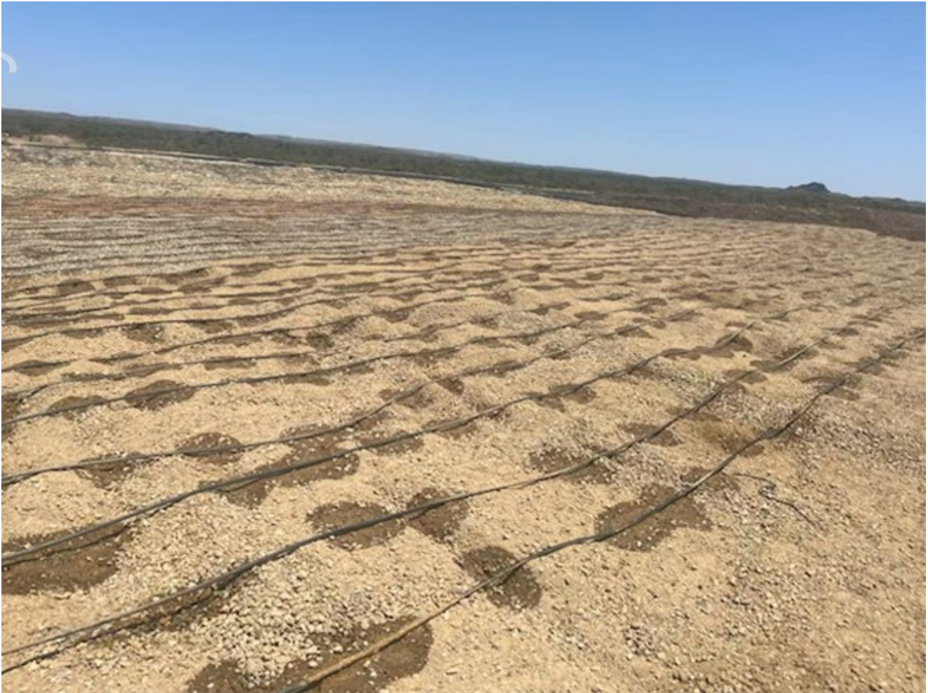
Figure 2. Leach pad 5 under irrigation on 8 October 2024.
