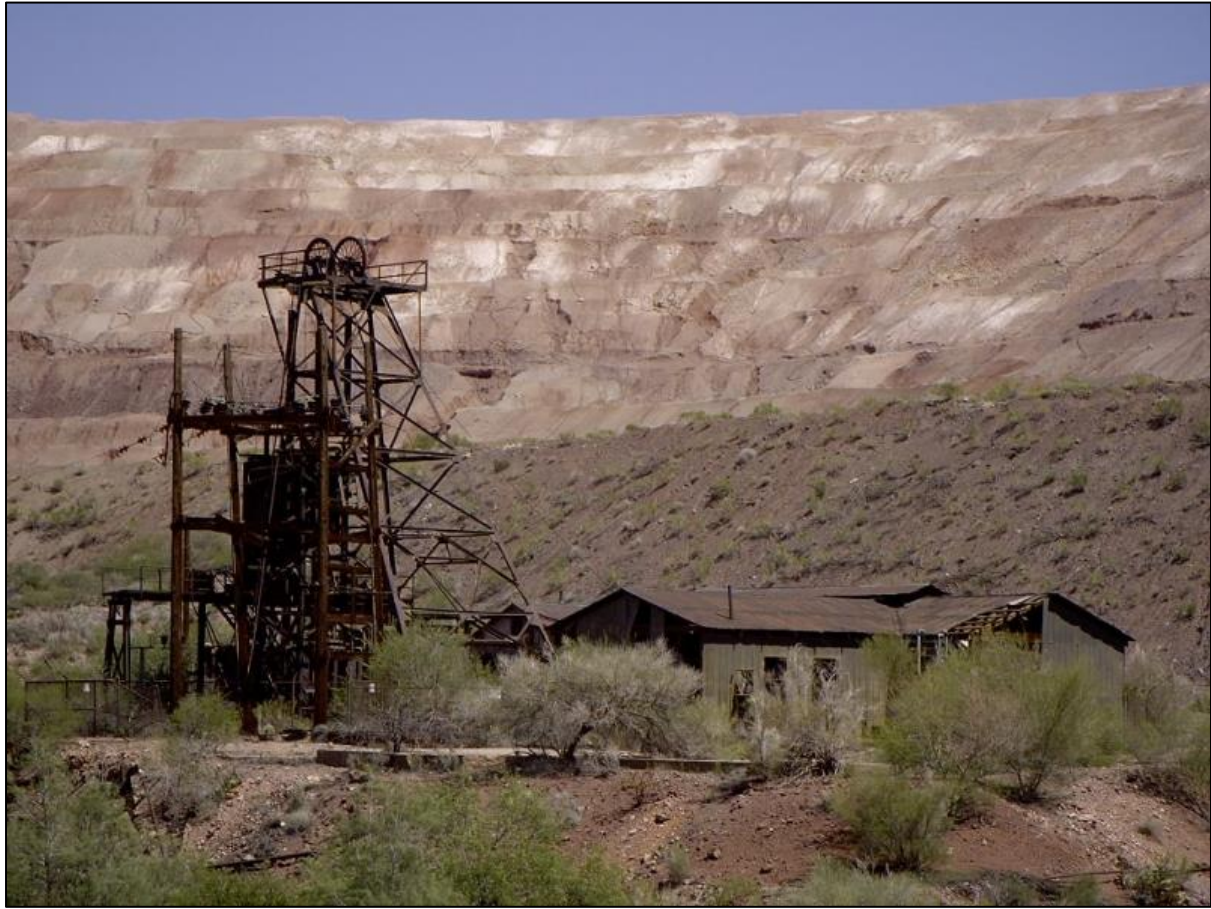
Figure 3: Headframe of the Tiger Mine, San Manuel, Arizona. Photo by Jon Spencer, 2010.
