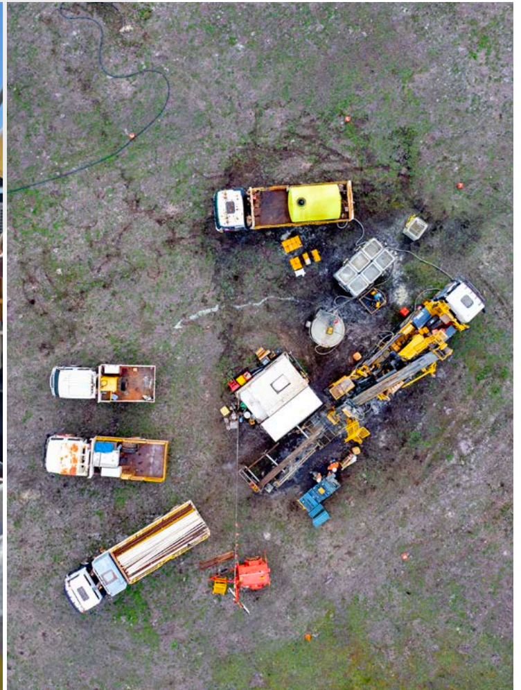
Figure 4: Drilling at the Springdale Graphite Project
