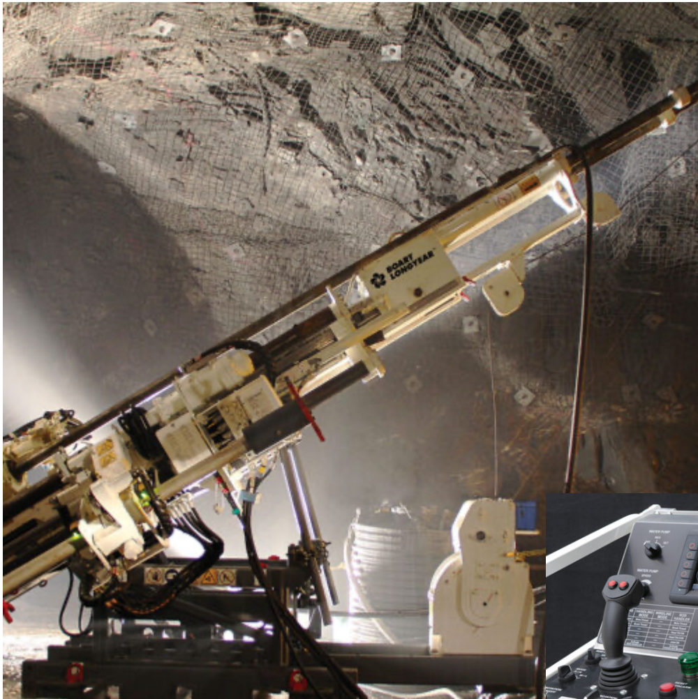
Figure 1: LM 90 Underground Drill Rig with Rod handler
