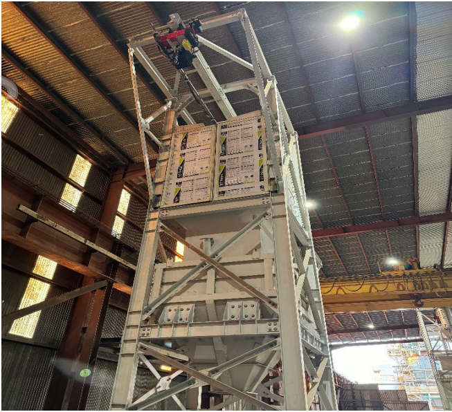
Ferrosilicon Bag Breaker erection (left) and Briquetting Ball Mill civil works (right)
