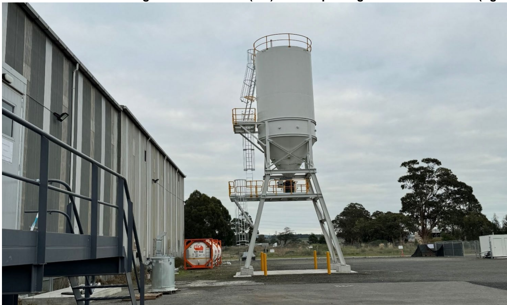
Supplementary Cementitious Material product (SCM) silo erection
