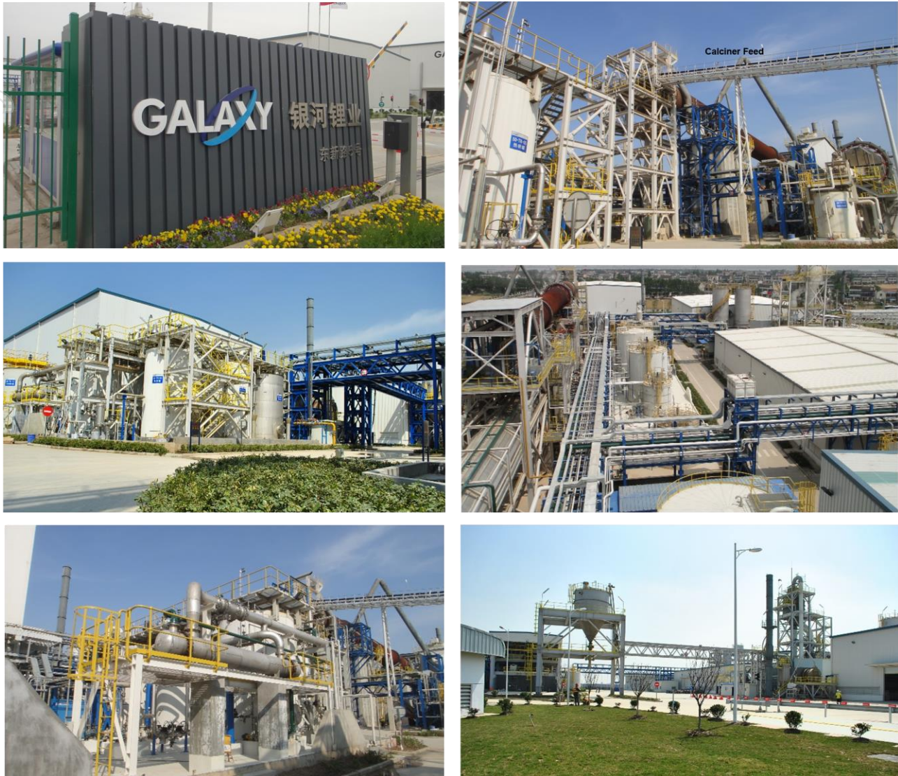
Figure 2: Galaxy Jiangsu Lithium Carbonate Plant
