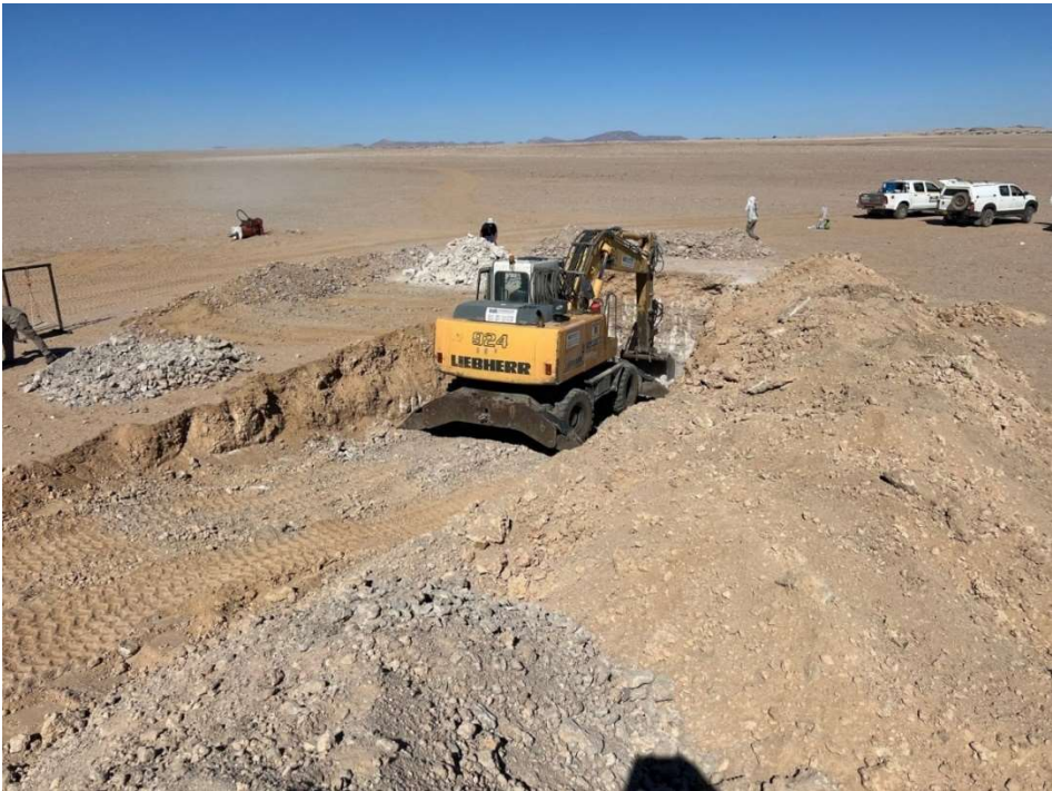
Figure 5 – Test Pit Excavation at Koppies Resource
