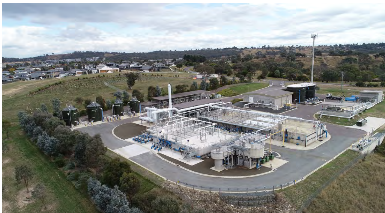
Googong Water Recycling Plant
