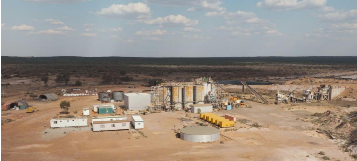
Figure 17 - Brightstar Processing Plant looking southeast
