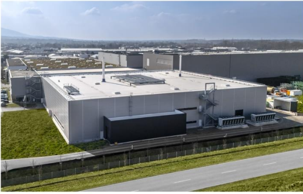
Figure 4 – Mercedes-Benz LiB Recycling Building, Kuppenheim Germany.
