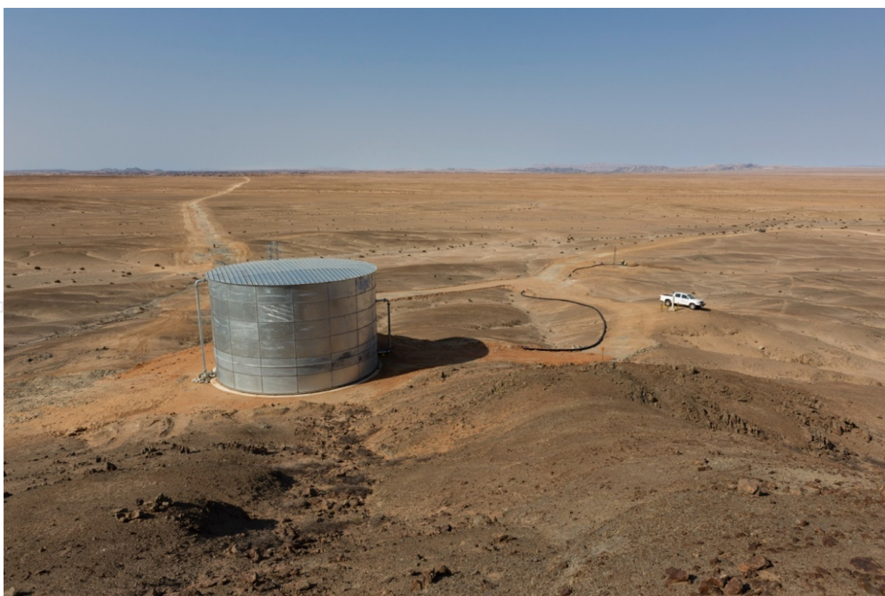
Figure 3: Completed construction water reservoir delivering 700m 3 storage volume
