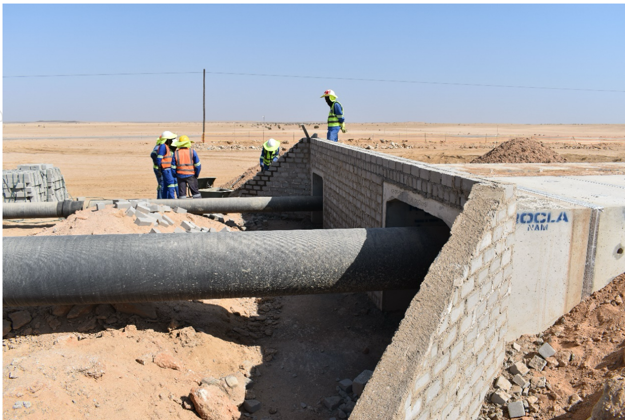
Figure 2: New culvert installed over the existing water supply pipelines
