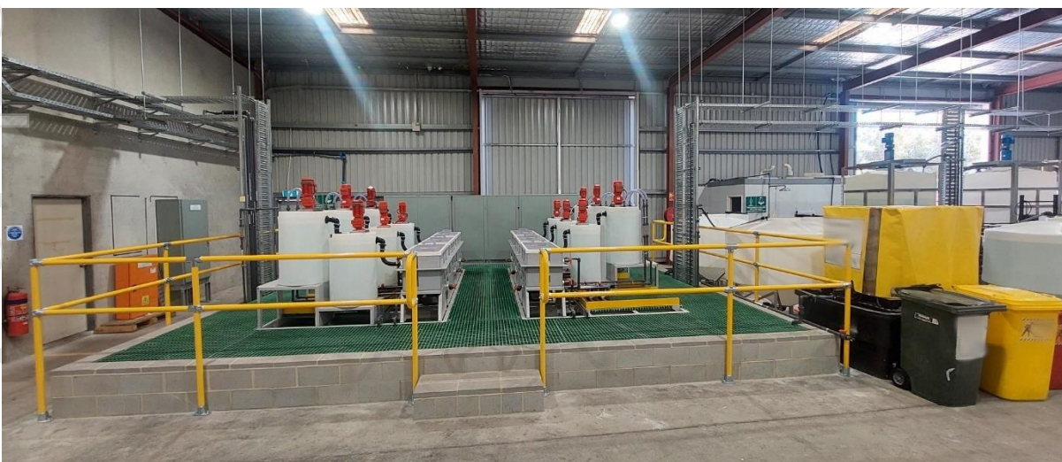
Figure 1 – ChemX HiPurA ® Solvent Extraction (SX) module completed, pending energisation infrastructure installation
