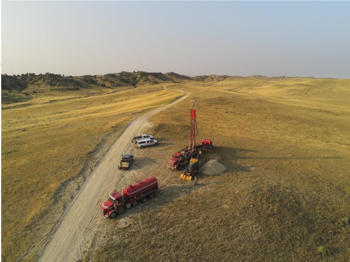
FIGURE 1. LO HERMA ISR URANIUM PROJECT DRILLING, POWDER RIVER BASIN, WY
