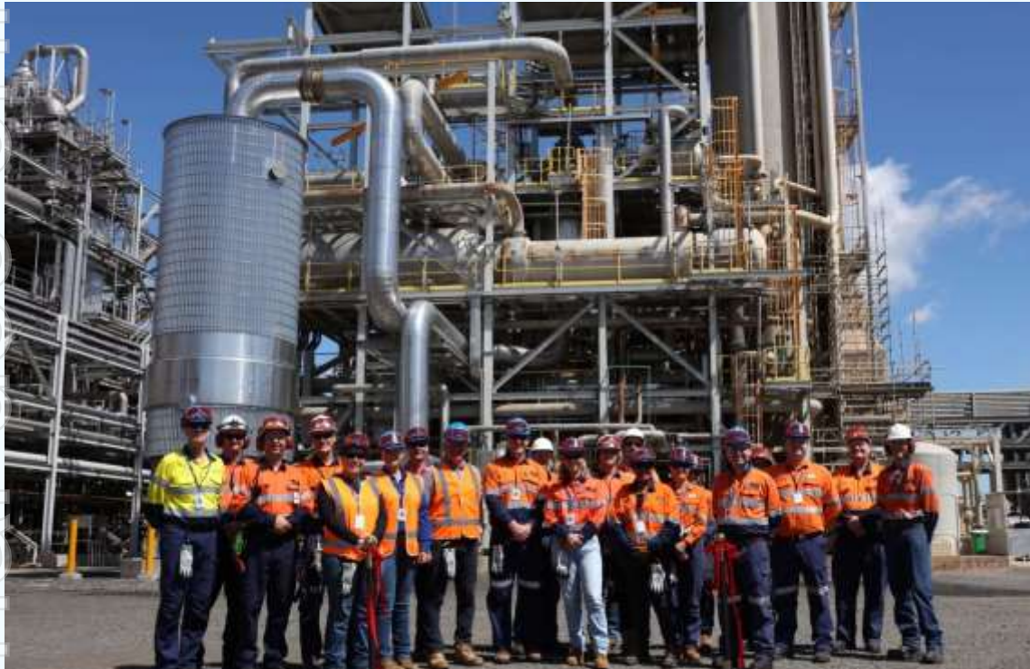
Official opening of Nitrous Oxide Plant, April 2024
