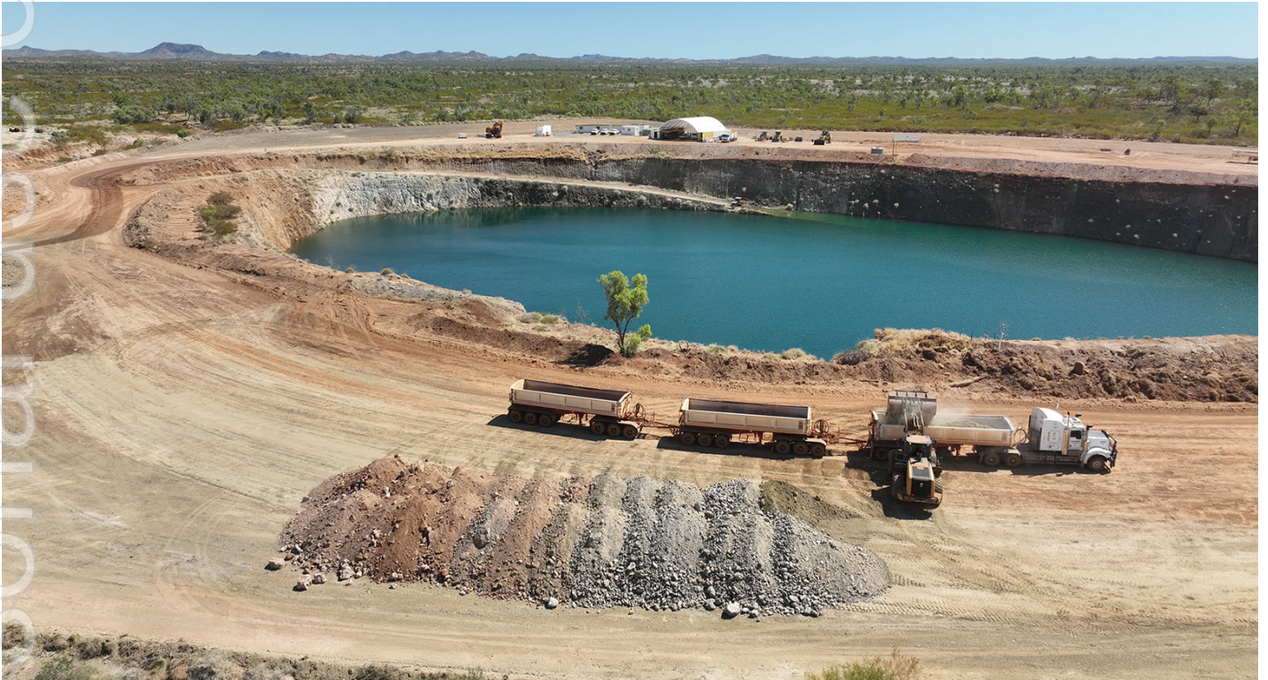
Figure 1. First Ore Haulage from Wallace North.
