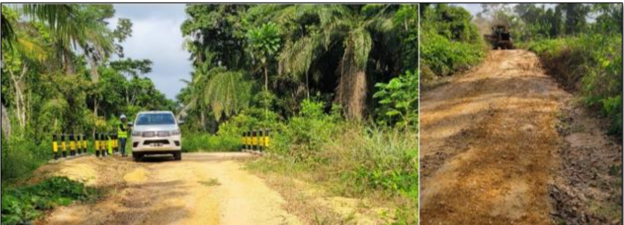
Figure 3 – Site access roads to the Cácata mine site being re-grated and upgraded.
