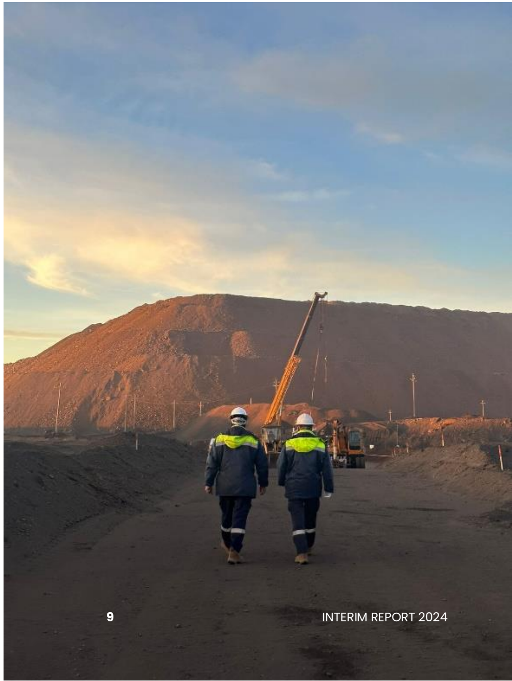
Preparation of drill pads for 2024 Pilot Well drilling
