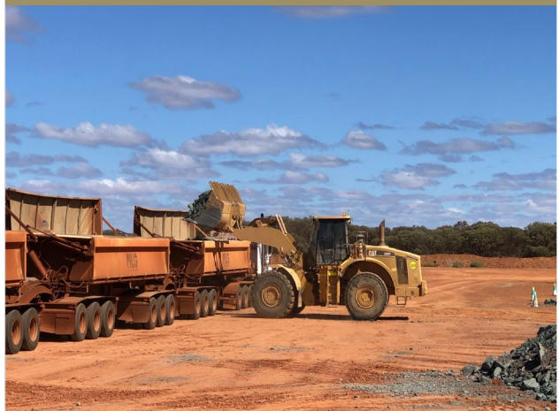
Ulysses underground - First ore haulage
