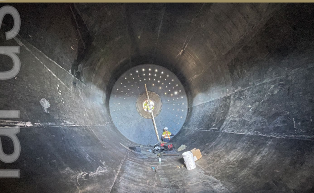
Laverton mill re-start - Ball mill relining
