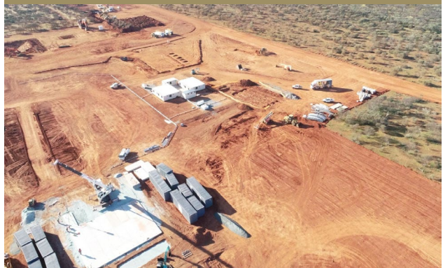
Hub open pit - Site infrastructure
