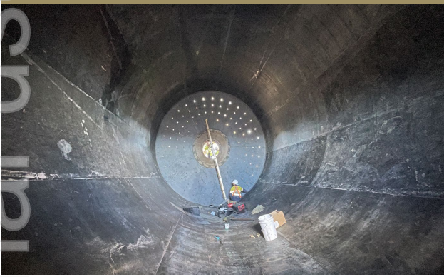
Laverton mill re-start - Ball mill relining
