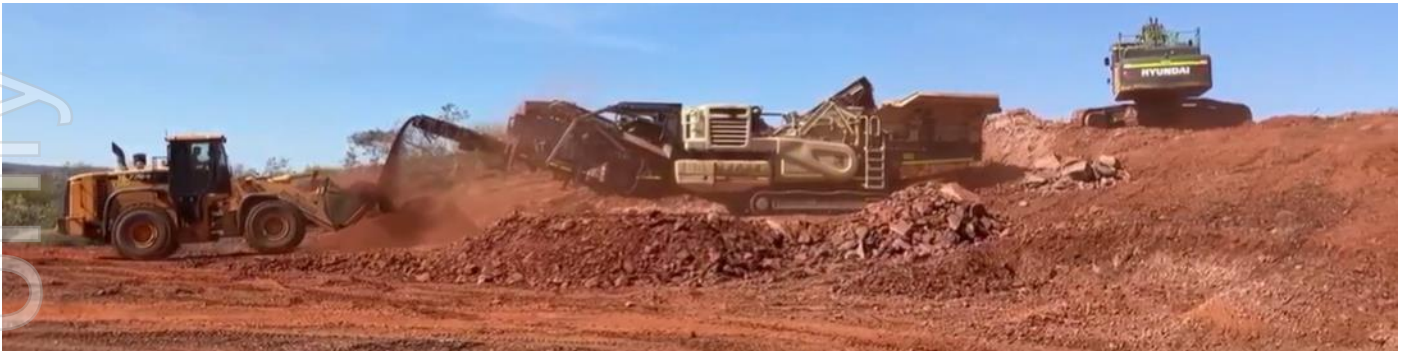
Figure 2: Commercial scale waste rock to road base product trial
