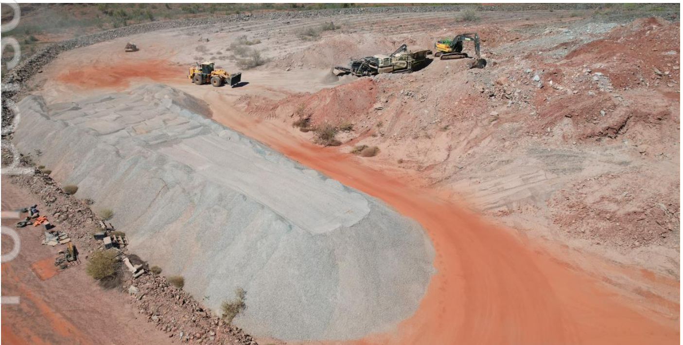
Figure 3: Commercial scale waste rock to road base product trial
