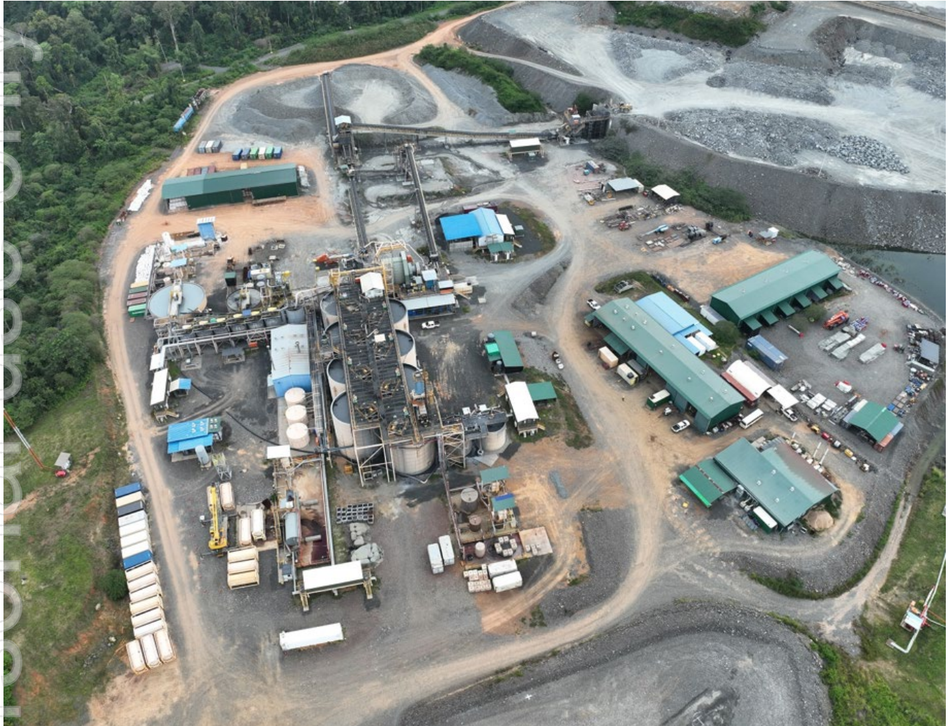
Figure 7 | Okvau Processing Plant
