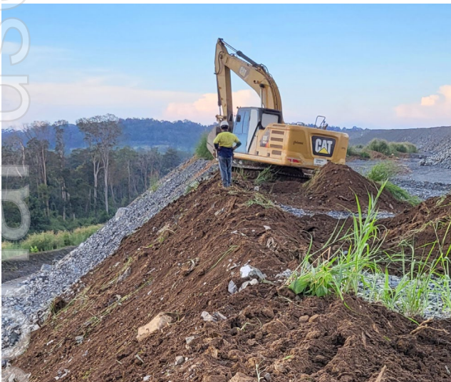
Figure 37 | Okvau batter/berm trial
