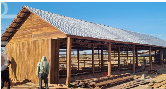
Figure 45 | New roof on school building
