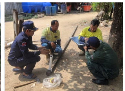
Figure 47 | Installing roadside lighting
