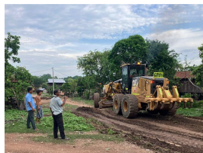
Figure 46 | Village road upgrades
