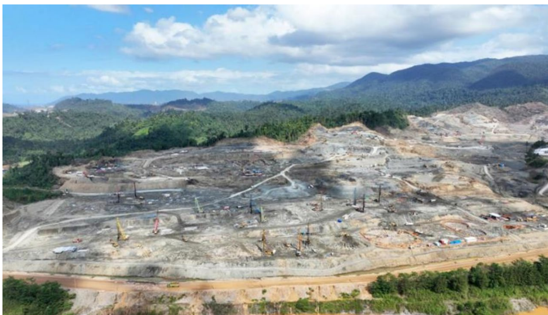
ENC Project under construction
