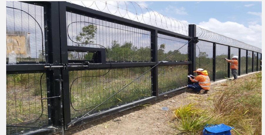
Security fence for rail corridor
