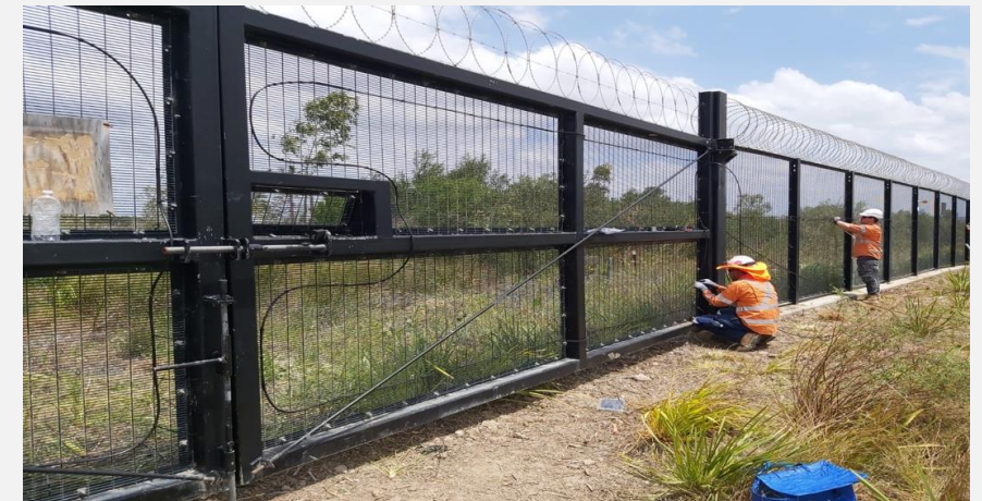
Security fence for rail corridor
