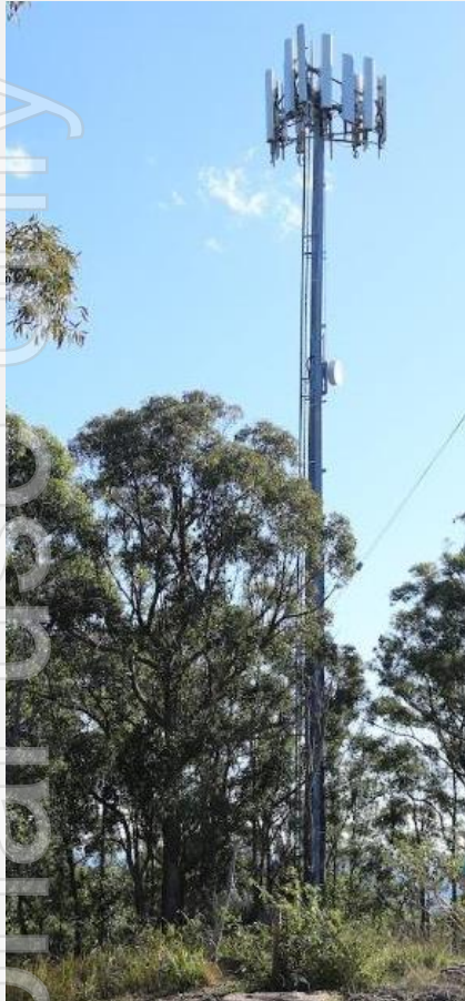
Securing mobile tower access
