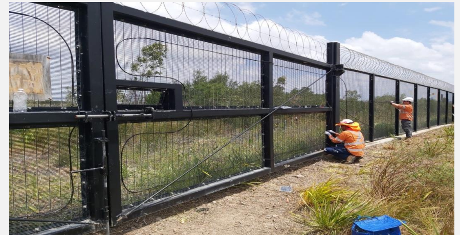
Security fence for rail corridor
