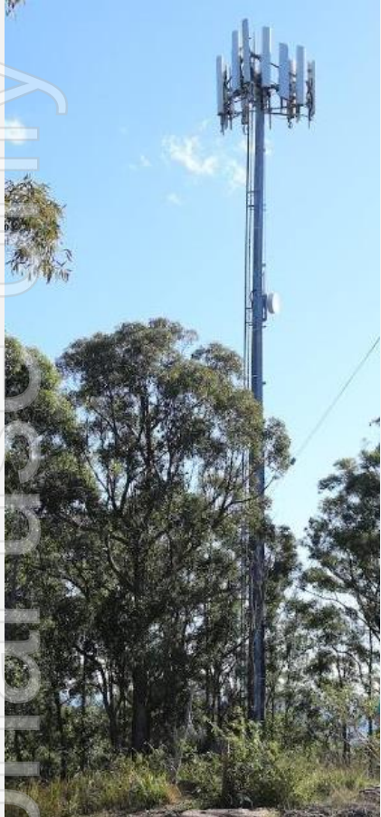
Securing mobile tower access
