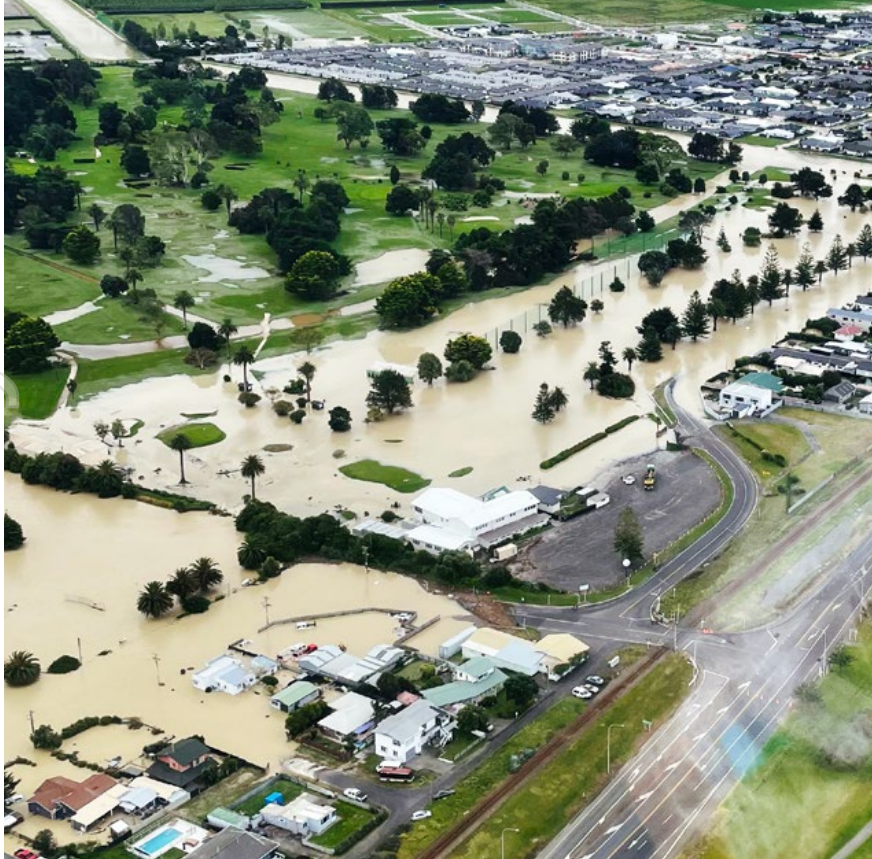
Flooding caused by Cyclone Gabrielle.
