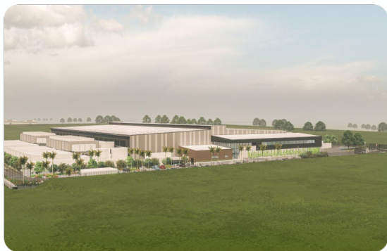
North Shore Data Centre
