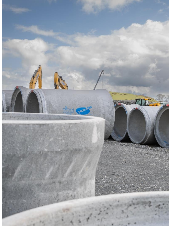
Stormwater pipes awaiting installation
