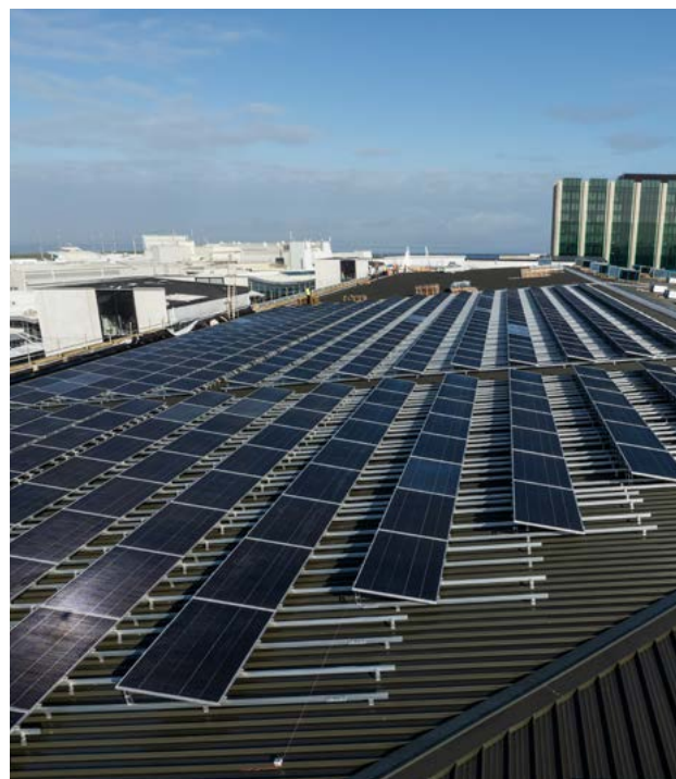
Rooftop solar panels on the Transport Hub
