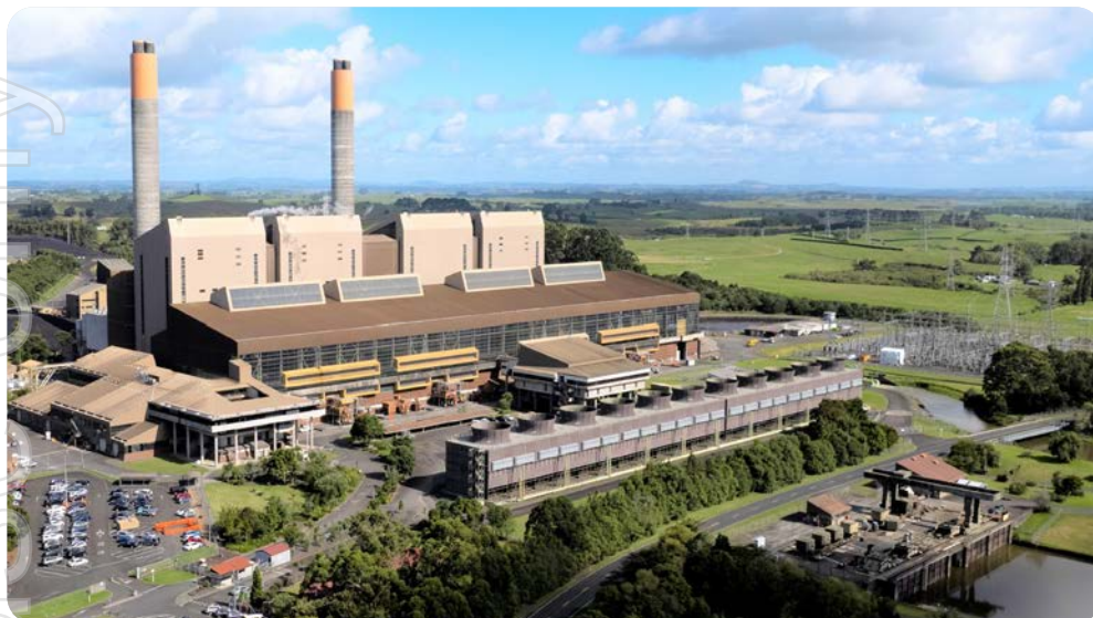
Huntly Power Station
