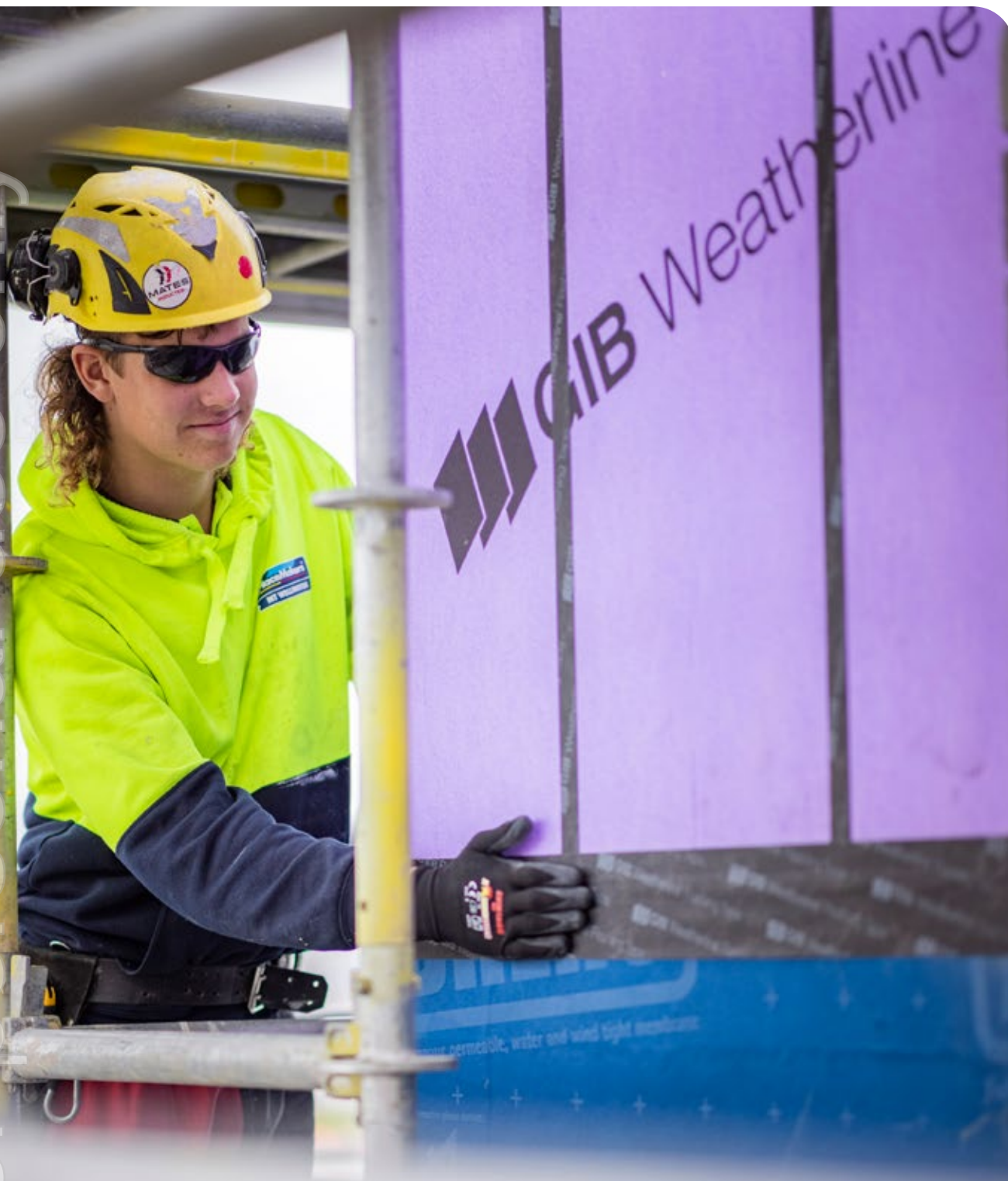
Subcontractor teams continue work on Fletcher Living's® Waiata Shores development.
