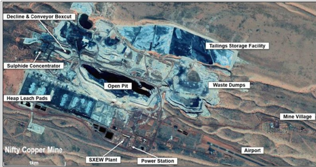
Figure 8-1: Nifty Minesite and key infrastructure (source: Nifty Copper SX-EW Restart Study)
