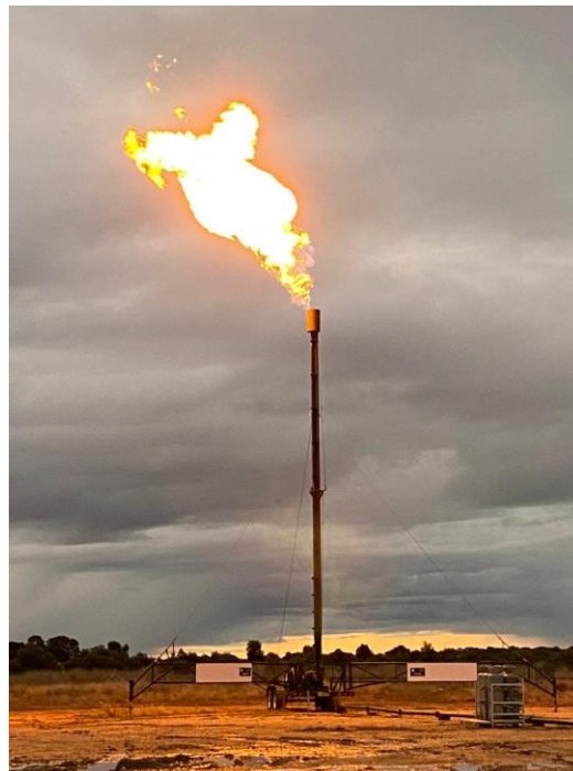
Gas flare of approximately 3 MMSCFPD from Daydream-2
