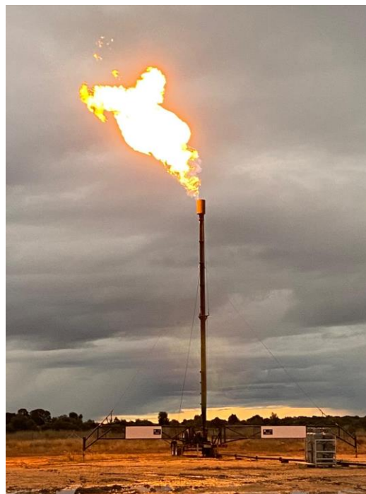
Gas flare of approximately 3 MMSCFPD from Daydream-2
