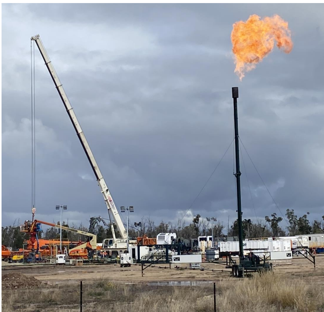
Daydream-2 wellsite during Lorelle Testing operation
