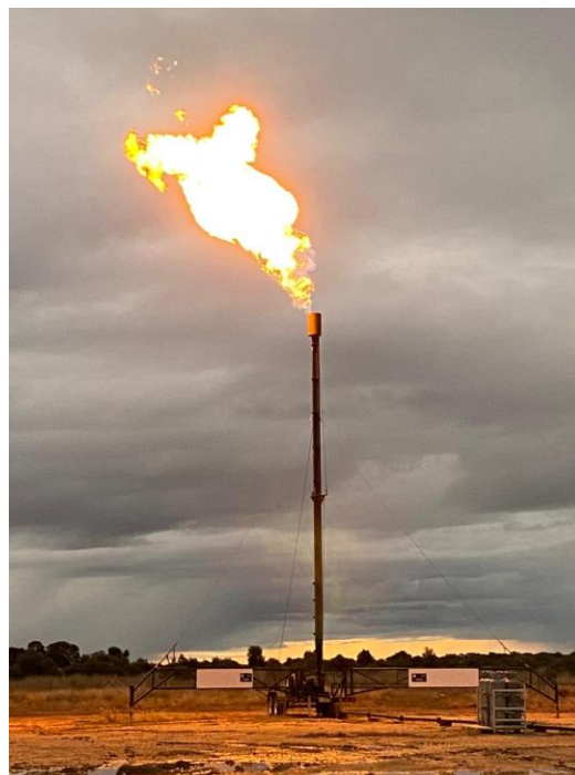
Gas flare of approximately 3 MMSCFPD from Daydream-2
