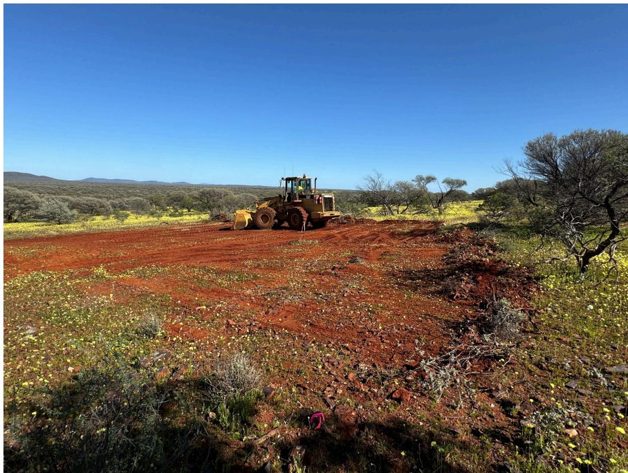
Figure 01: Earthworks commencing at the Remorse Target
