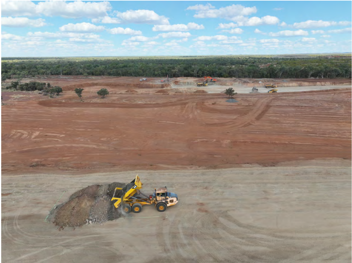
Figure 2. First Ore delivered to Wallace North RoM Pad.
