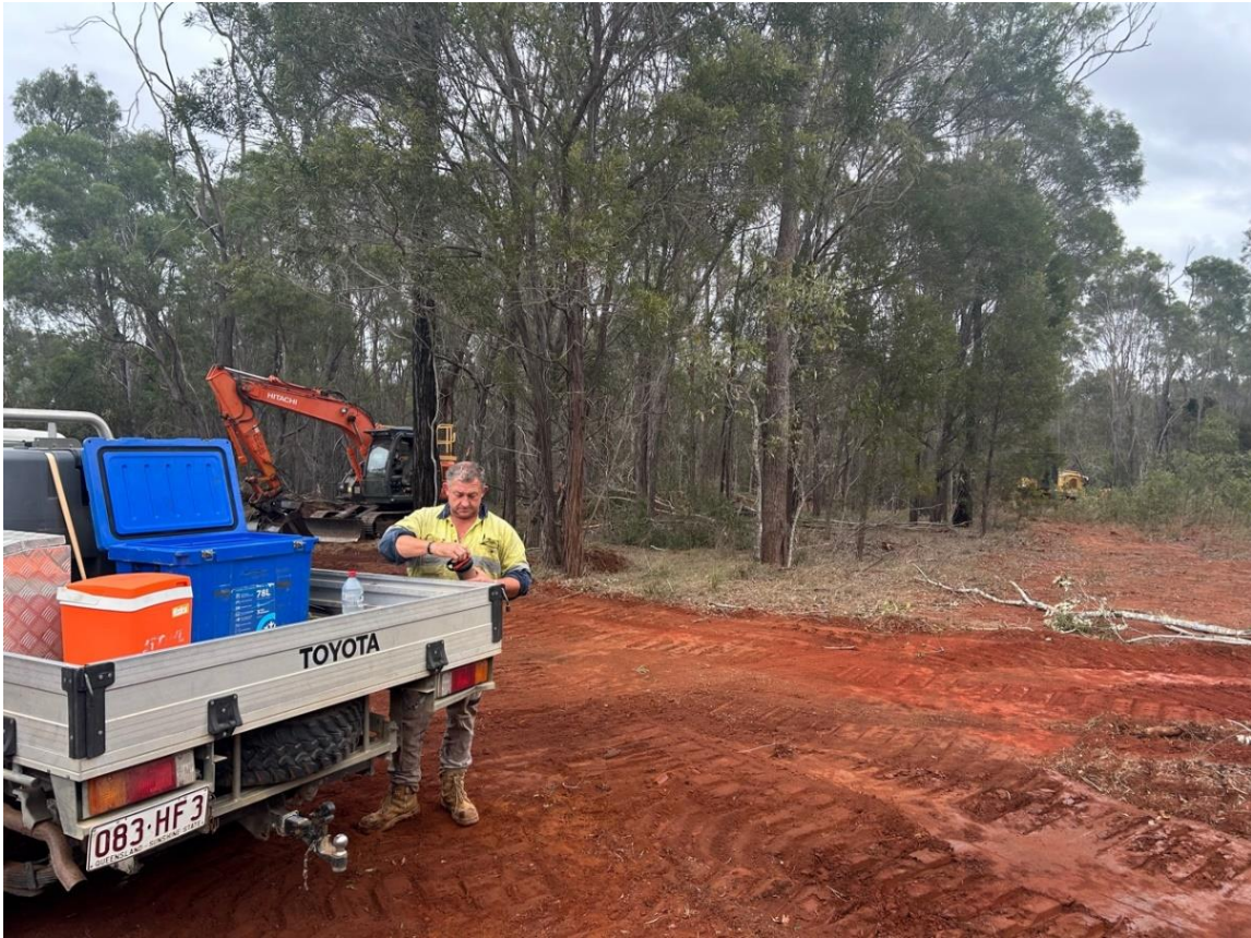
Figure 3: Develin Creek drill pad preparation in progress.
