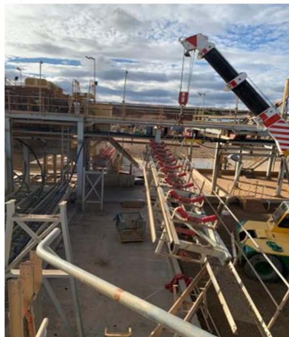
Figure 2: Photos showing dismantling of the 400kW ball mill and associated processing infrastructure at Wonawinta in preparation for its relocation to Mt Boppy.
