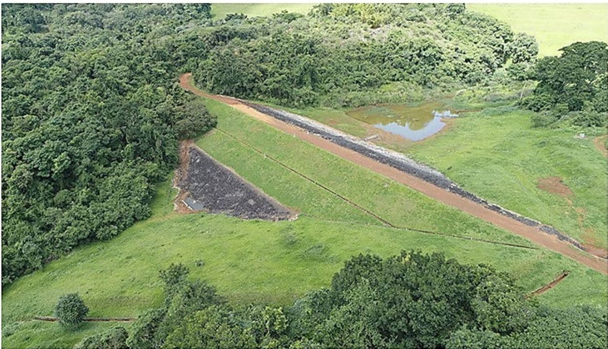
Figure 2 – photo of Dam D. Source: https://cbmm.com/en/our-company/our-dams
