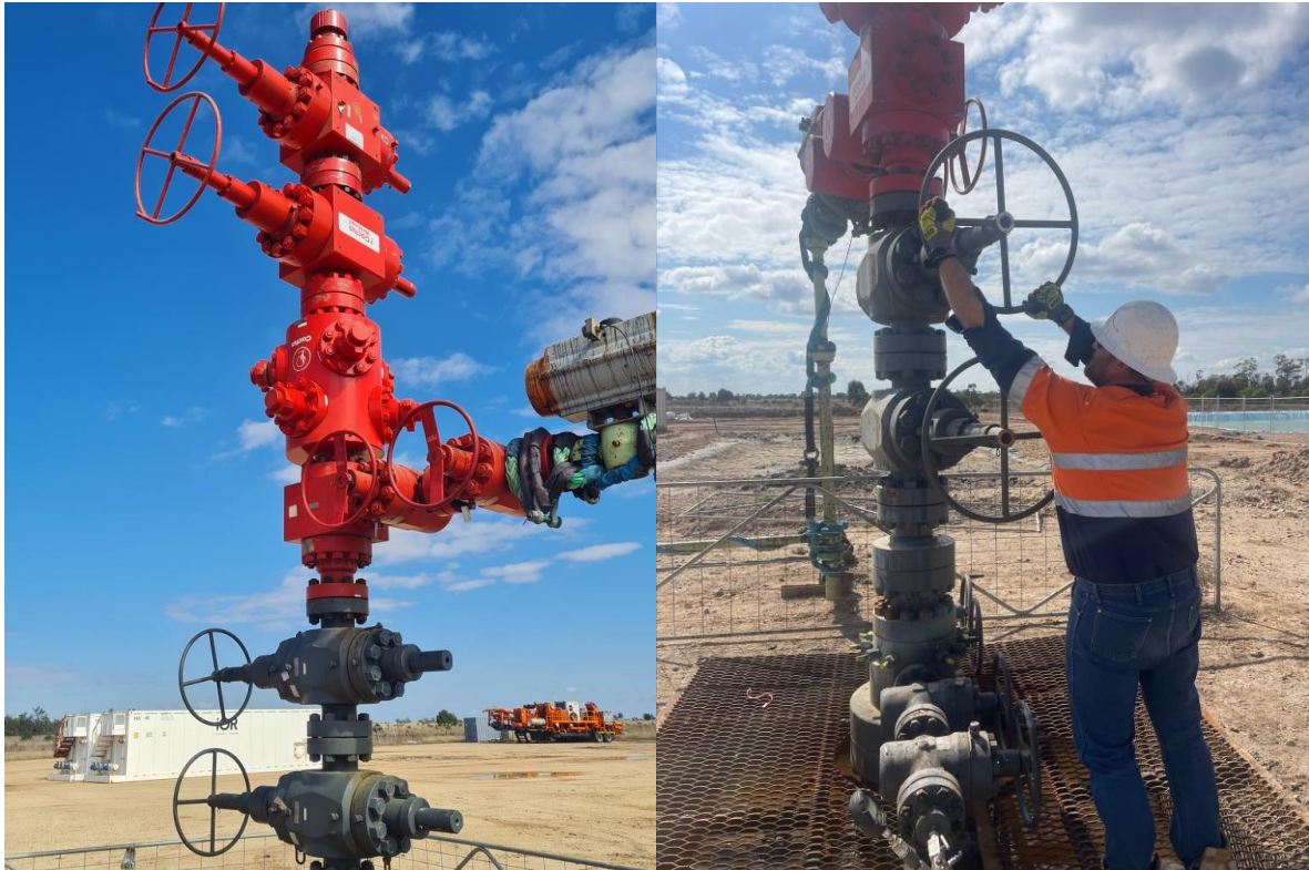
Servicing of well head at Daydream-2
