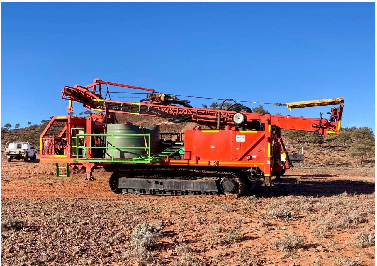
Figure 1: Diamond drill rig at Bald Hill yesterday afternoon (7/8/2024)
