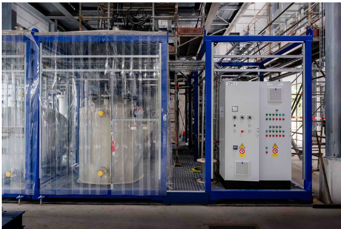
Figure 5: Crystalliser Package
