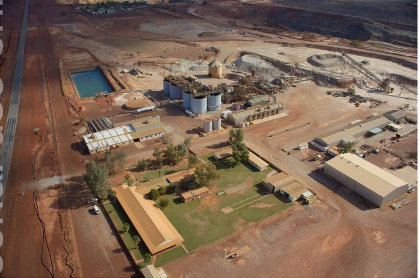
Figure 8. Westgold Bluebird Mill and Processing Facility
