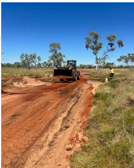
Figure 1: Kundat Djaru (Ringer Soak) Floodway Crossing repairs
