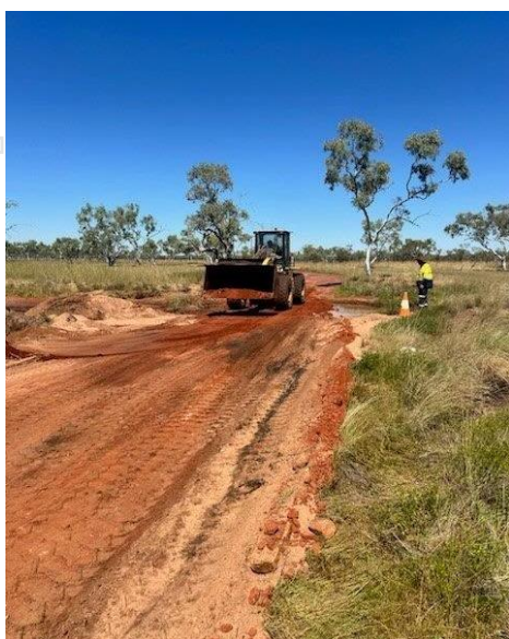
Figure 1: Kundat Djaru (Ringer Soak) Floodway Crossing repairs
