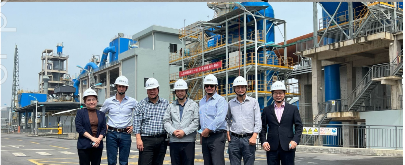
The Company inspects an operational lithium refinery within the Sichuan province, China
