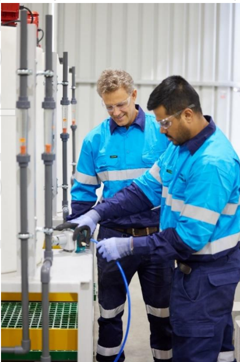
Figure 2 - ChemX Team actively plumbing key reagent delivery systems to the unique HiPurA® SX Circuit
