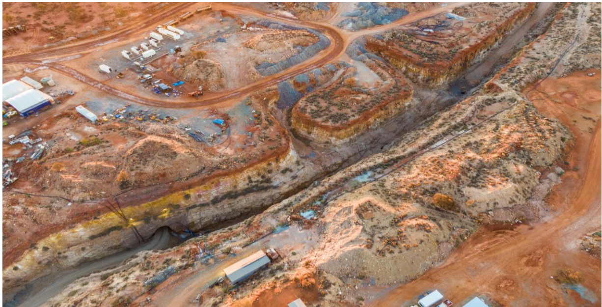
Figure 6 - Second Fortune underground portal
