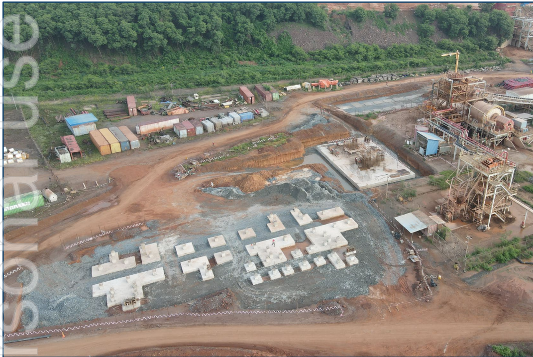
Ball mill and flotation area foundations
