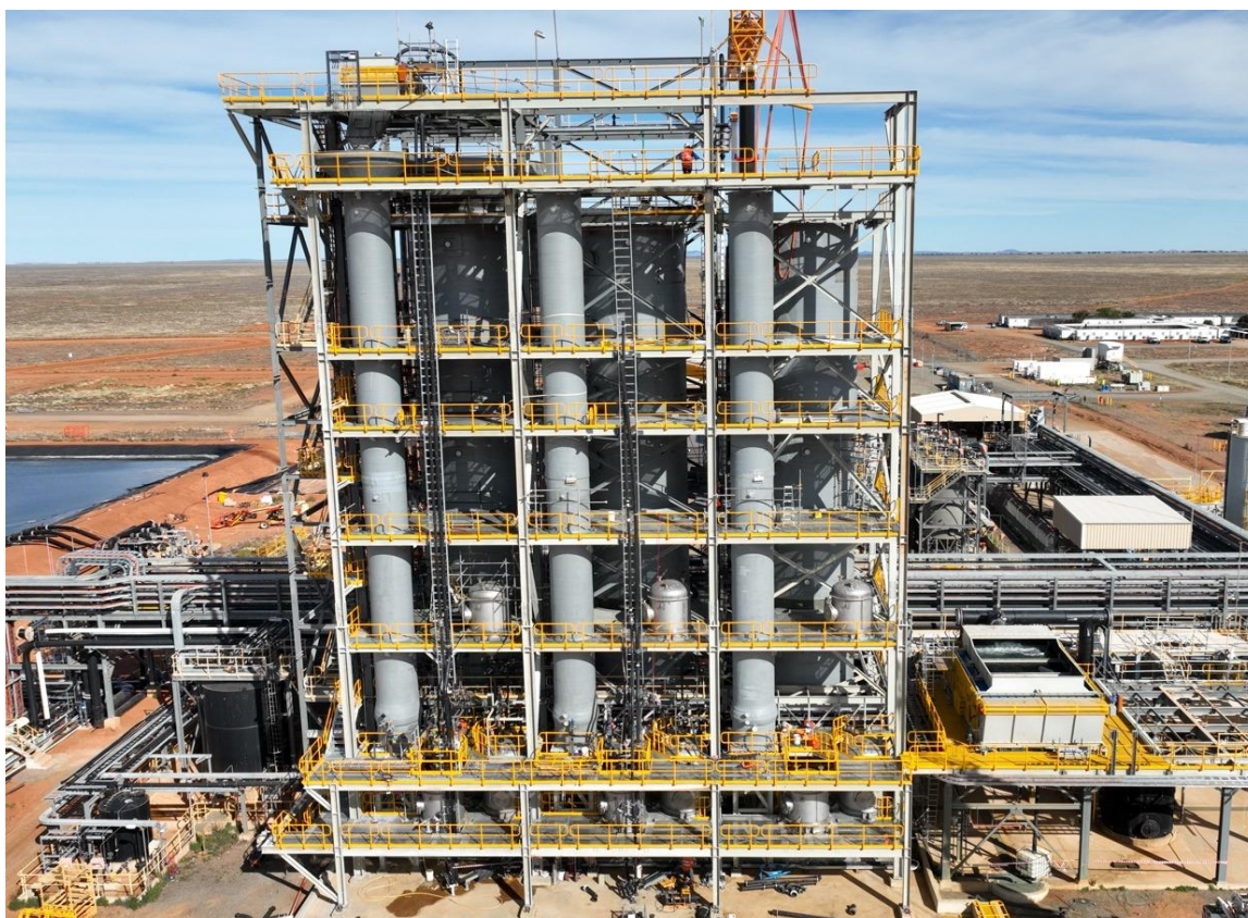
Figure 1: Construction of NIMCIX columns 2 and 3 nearing completion
