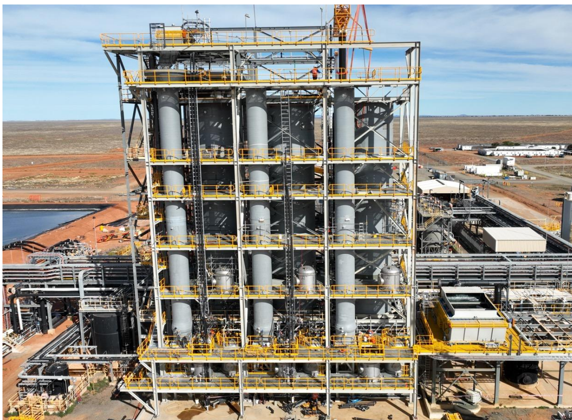
Figure 1: Construction of NIMCIX columns 2 and 3 nearing completion
